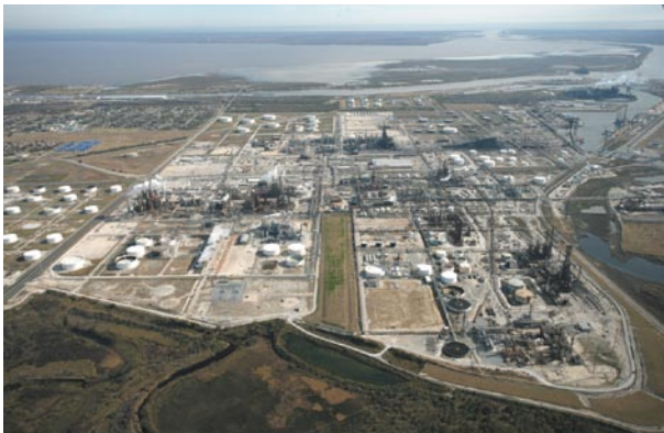
Figure 5. Aerial view of Port Arthur 1 and 2.
