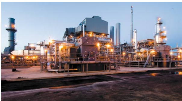
Figure 3. The hydrogen production facility at Convent, Louisiana.
